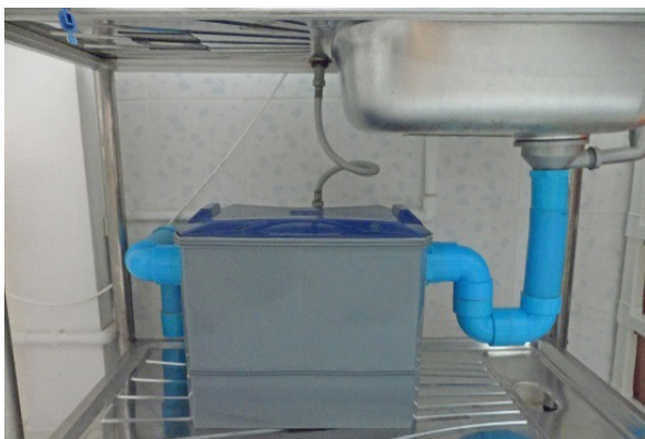
(a) Examples of grease traps Source: https://pantip.com/topic/35866812
