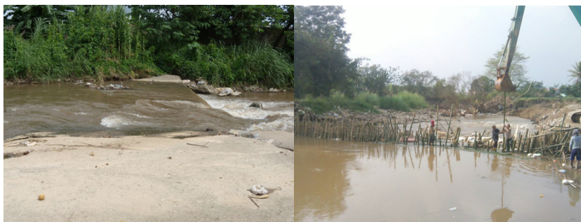
Figure 2 (left) Fai Muang Ngam rock-fill weir for Right Main Canal (RMC) 3, probably taken in March 2007; (right) temporal, bamboo weirs, taken in April 2018
