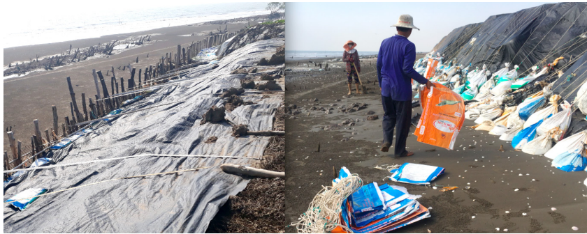
Figure 4 Local farmers renovating their sandbag revetment system (photo taken on 6 June 2020)
