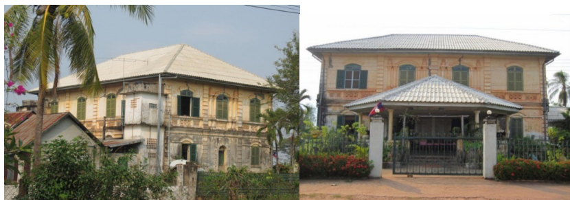
Figure 9 The front and side of the residence of Chao Ratsadanay in Champasak. Modern materials and designs are incorporated and vents have been added at the top of windows to facilitate air flow.
