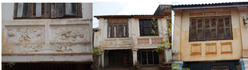
Figure 6 Shophouses during the colonial period are believed to have been the dwellings of Vietnamese migrants. Decorative stucco and numbers are usually found in shophouses in the town of Pakse.
