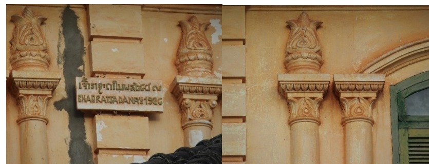
Figure 10 The heads of the decorative columns reflect valuable historic images, cultural acceptance, adjustment between the western and local style, and the use of cement, a modern material.
