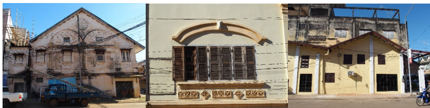
Figure 4 The patterns of western-style buildings are altered to suit the local climate by adding vents and windows to facilitate air flow
