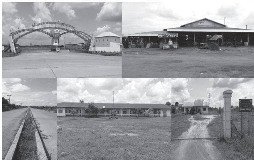
Figure 4 The infrastructure in the resettled village
