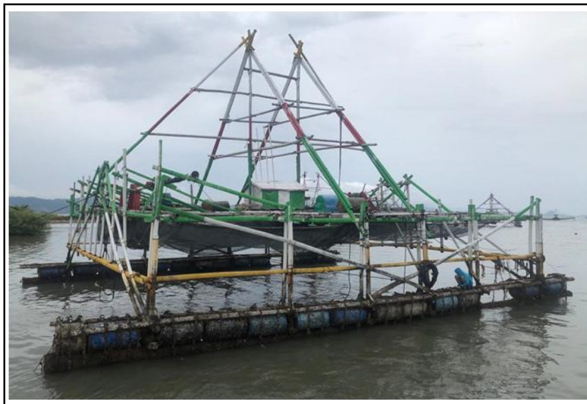
Figure 2: Construction of Bagan in Lampung Bay
