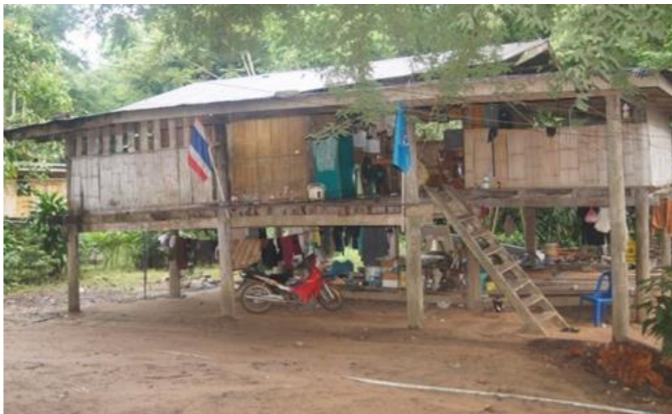
Picture 1: Example of the Characteristics of House Construction in the Karen Community, Ban Yang Hak
