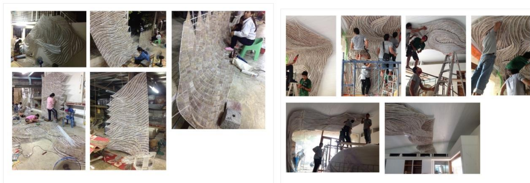
Figure 6 Project progress and Installation of work
