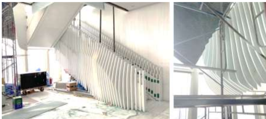
Figure 11: Process for Installing Parametric Stair
