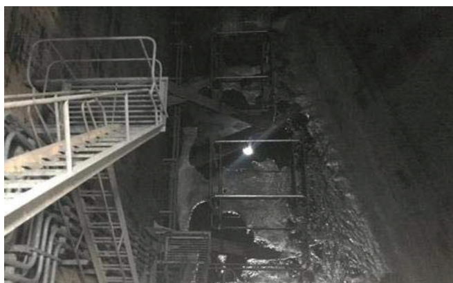
Figure 6 Sludge in the cargo tank
